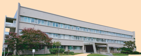
Administrative Office Bldg.
