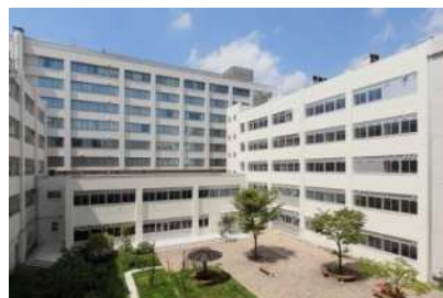
(本道)臨床校舎(北)改修
